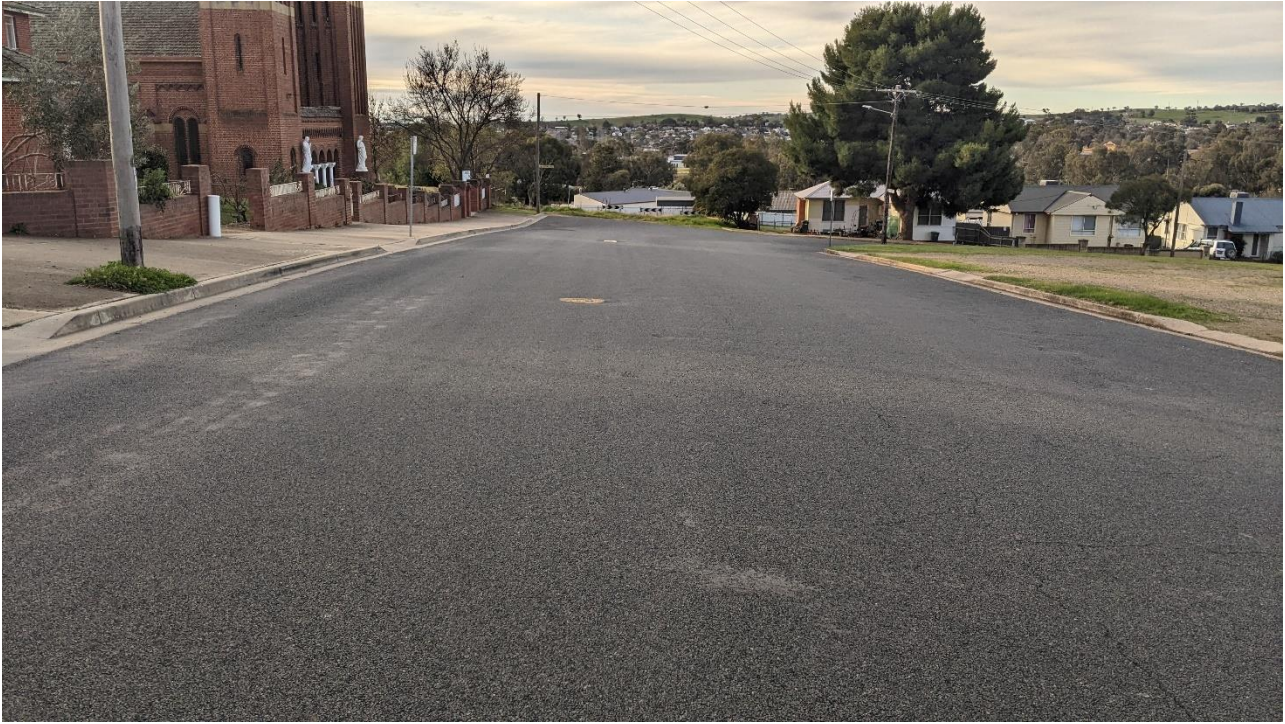
Figure 5: View looking north along Kitchener St adjacent to school bus zone
